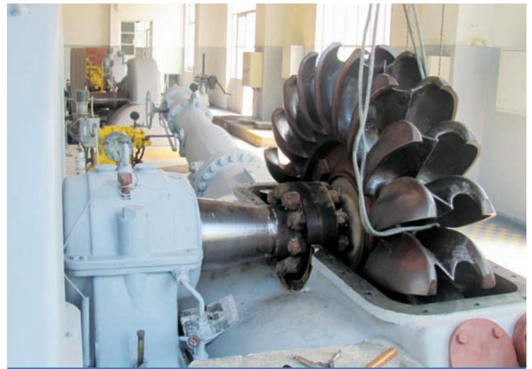
The Pelton wheel being welded at one of the turbines at the Rachmaya hydropower plant
