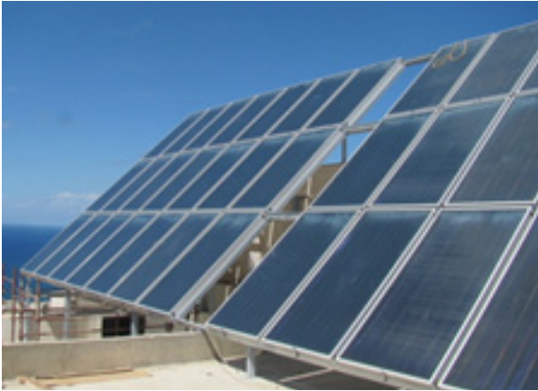
Figure 12: Keserwan Public Hospital - SWH roof structure installation (source: Cedro)
