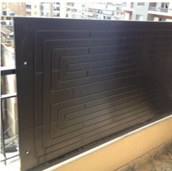
Figure 13: Solar thermodynamics panel
