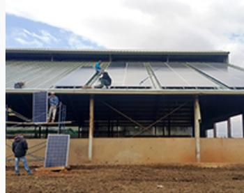
Following the competitive bidding process, Phoenix was awarded the implementation of a 214 KWp PV-diesel hybrid system at Libanlait in the Bekaa. Installation of the system on the farm side of the facility started early this year and is expected to be completed by end of April. The project co-benefit will be providing vital extra insulation for the farm shed while producing green energy.
